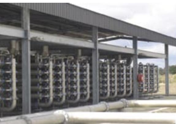
Figure 7 Membrane filtration bank for recycling water at South East Melbourne
