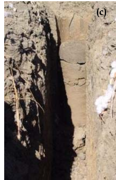
Fig. 4 (a) Lowering the lysimeter back down the hole. (b) The lysimeter in place with plumbed drainage line extending back to the edge of the field (towards the camera). (c), the intact soil cores placed in original order on top of the lysimeter, before the hole and access trench is in
