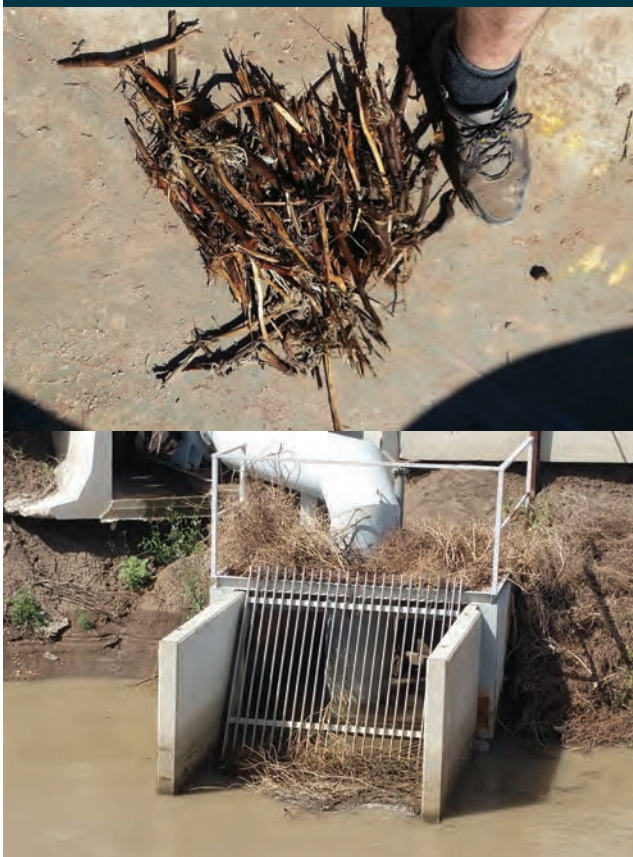
FIGURE 9.2 Cotton trash can reduce pump performance by up to 30%. © Phil Szabo
