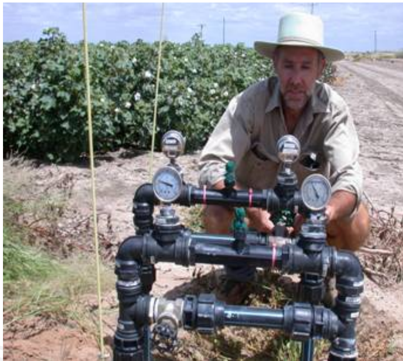
Photo 15 RWUE3 officer Lance Pendergast inspects oxygation equipment at drip irrigation demonstration
