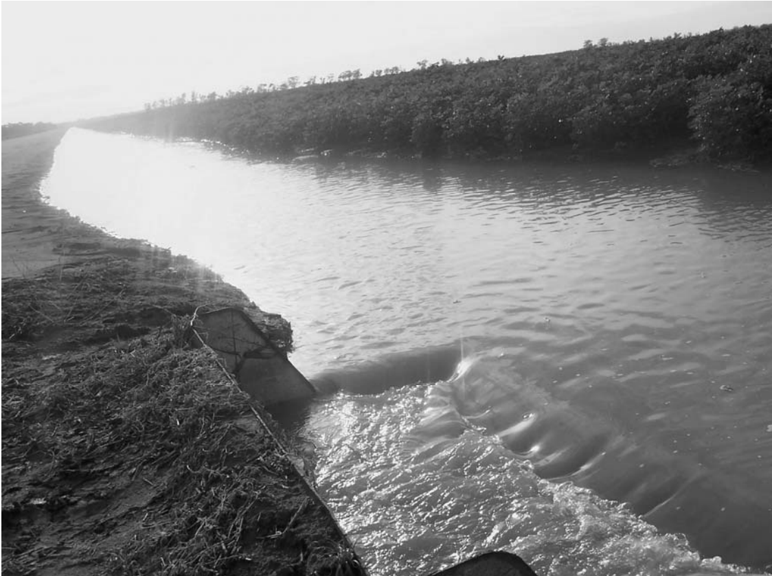
Figure 4 – Tail drain of “Willawah” field 3
