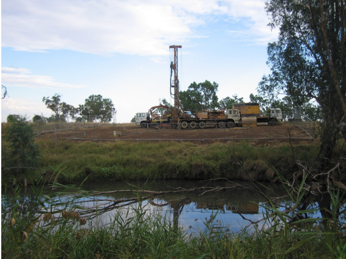
Figure 13: Drilling at Elfin's Crossing
