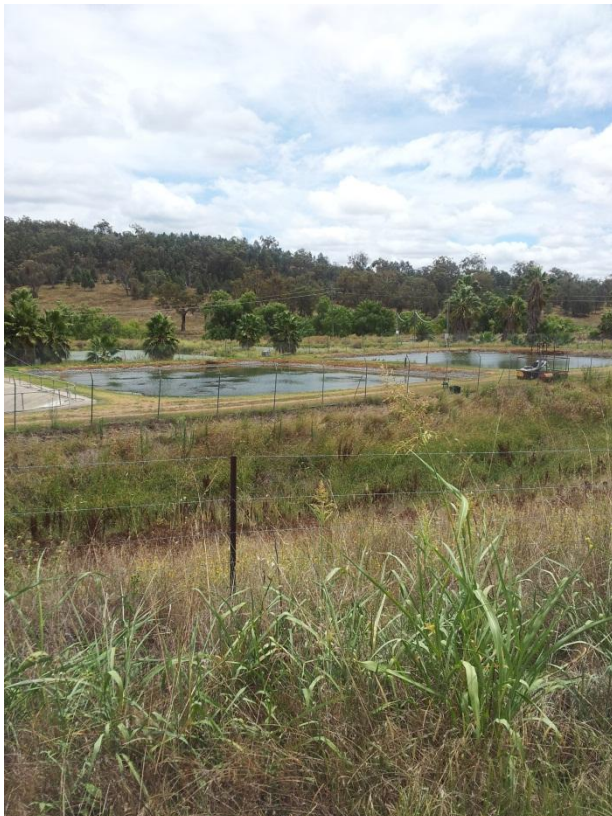
Photo 2: Waste Treatment plant at Quirindi
