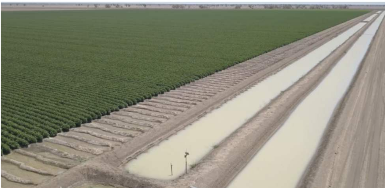
Figure 2: A small pipe through the bank, or bankless system used to irrigate cotton at “Waverley” Wee Waa
