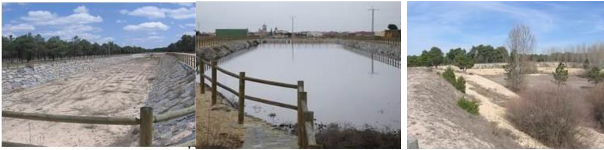
Figure 11 Gomezserracin infiltration pond in dry and wet season, and sandpit reused as infiltration pond.
