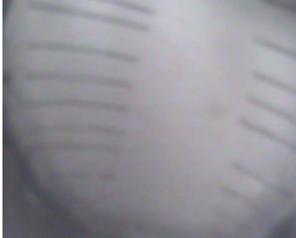
42220032 - Slots in casing (29.8 m - 30.5 m).
