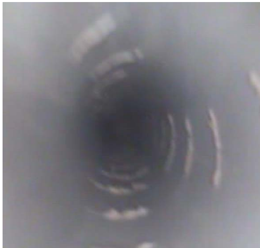
42220056 - Slots in casing (17.1 - 18.1 m).
