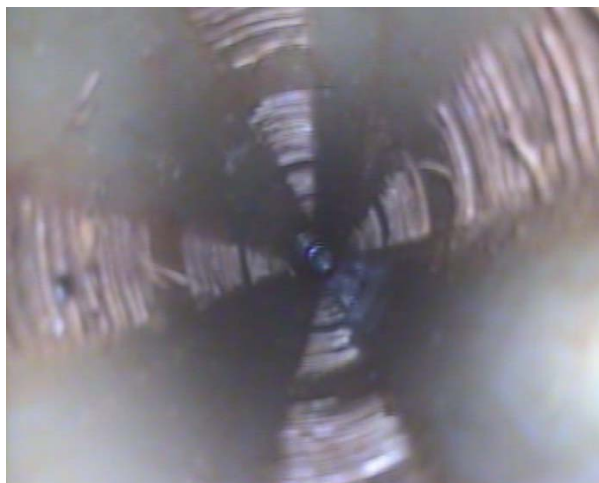
42220033 - Slots in casing (at 29.8 m – 30.47 m).
