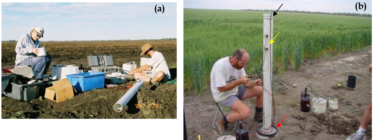
Fig. 5 (a) Building the lysimeter-related apparatus in the field. (b) Plumbing the vacuum tower that supplies the vacuum to the lysimeter. Arrowed are the water reservoir (red), reed switches (yellow) and vacuum supply line (black). The electrical pump (Fig. 6) draws the water up past the lower reed switch, to the upper switch that triggers the pump “off” – creating a vacuum as the water drops back down the column. Passing the lower reed switch, the pump is switched back “on” to again raise the water in the tower.
