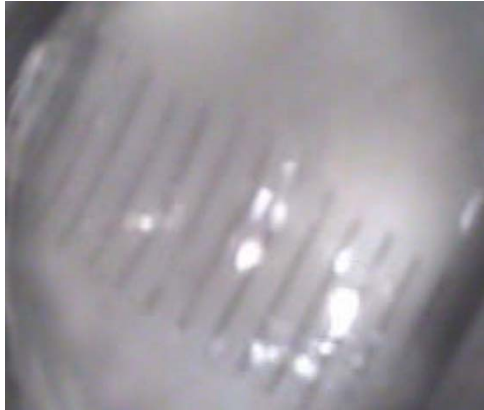
42220034 - Slots in casing (at 20.66 m - 21.33 m)
