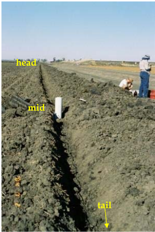
Fig. 7 Trenches to carry the vacuum line (a) along the edge of the field to link each of the three lysimeters, located at the head ditch, mid-field and tail ditch locations, and (b) from each lysimeter out to the edge of the field.
