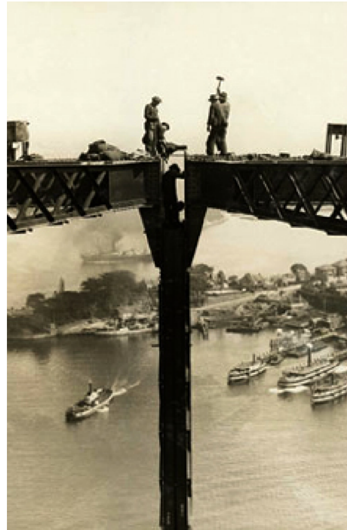
Builders, Sydney Harbour Bridge
