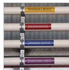
Figure 3. PVC pipes taking separate dissolved fertilisers to the pycnometer point.
