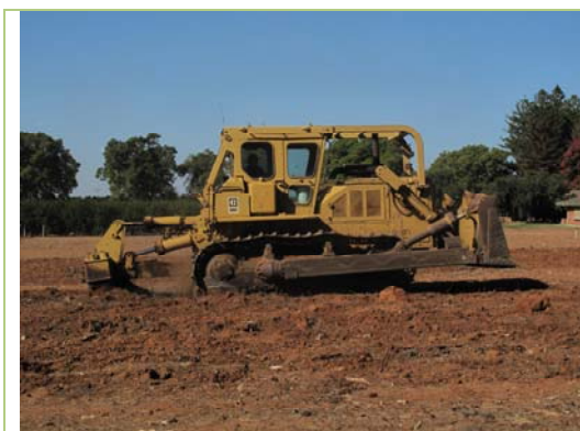
Figure 53 Trial site being ripped to 1.2 m following removal of tree stumps
