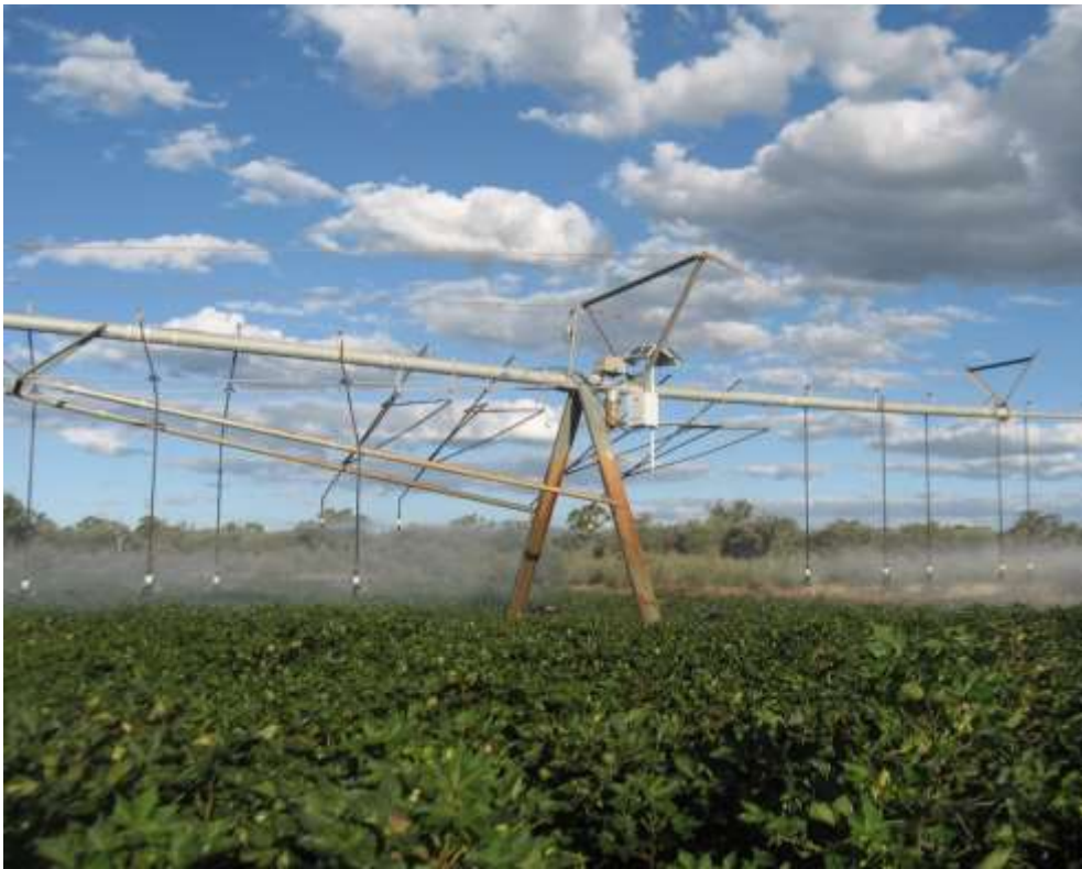
Figure 2 Installed PIMS unit on a Centre Pivot
