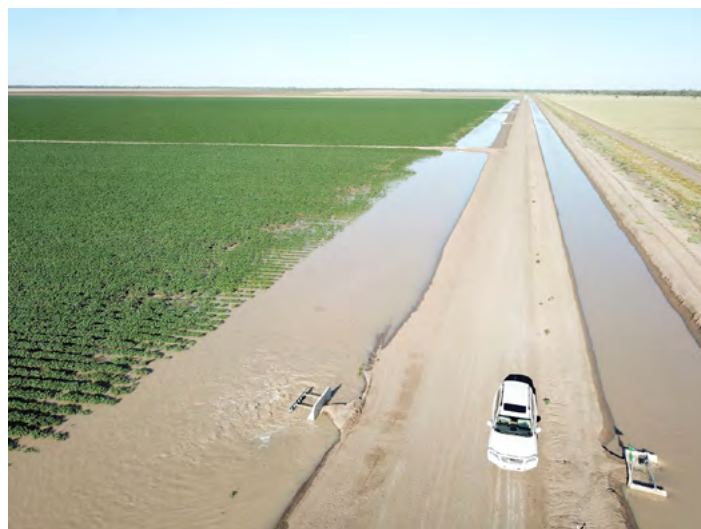
Figure 1: Pipe through the bank is one example of a siphonless layout.
