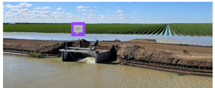
Figure 3: Pipe through the Bank is an example of a siphonless layout that has evolved as cotton growers adapt layouts to improve productivity and resource efficiency.
