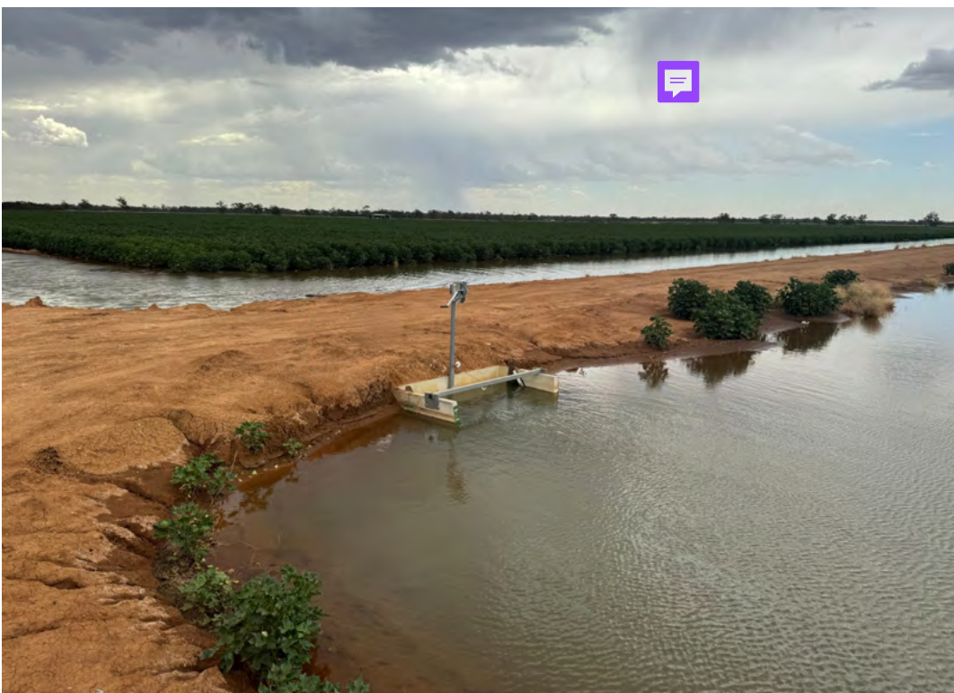
Figure 11: In a Rollover Basin, the furrow direction follows the slope of the landscape and machinery can 'rollover' the bankless channel into the next basin of the same field. In this image the road is between two basins of the same field, with a bankless channel on both sides of the road. The bankless side channel connects the basins via a pipe under the road.
