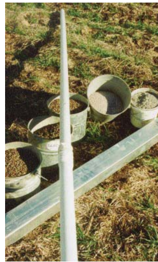
Figure 3 – Materials to install a shallow monitoring piezometer
