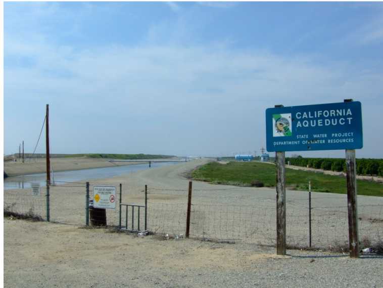
Figure 14 The California Aqueduct.
