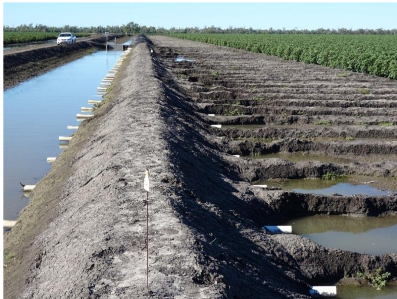
The Redmill site viewed from downstream after the flow had been shut off
