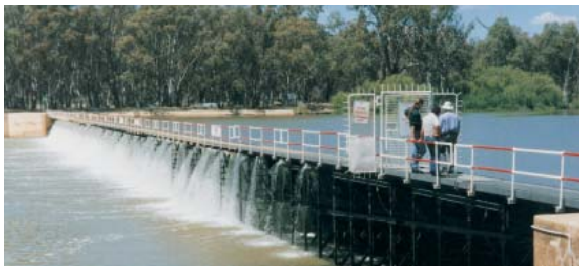
A large weir without a fishway on the River Murray, South Australia.
