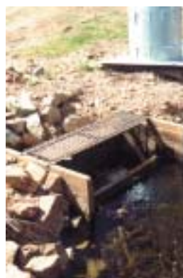
Photo 1: Drop board flow culvert blockage at outflow of deepwater lagoon. These types of structures limit the capacity of many species to move between habitat reaches.
