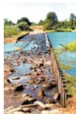
Photo 2: Weir on Haughton River. Design elements intended to act as flow energy baffles actually facilitate upstream fish passage around this weir under certain flow conditions.
