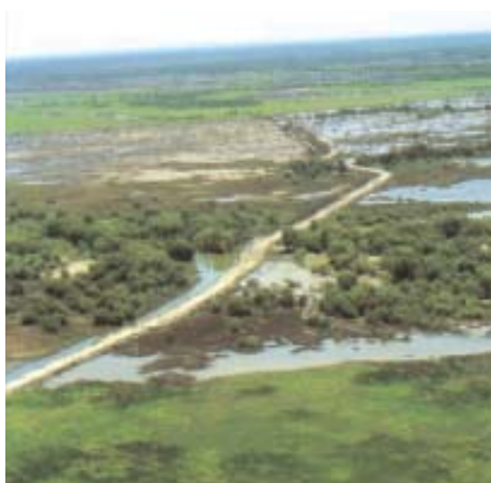
This photo shows a bund wall situated on the west of Tommycut Creek.
