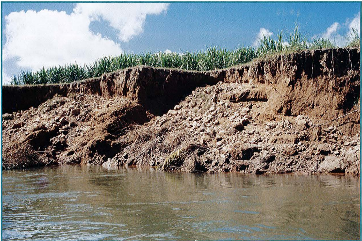
The removal of riparian vegetation has resulted in streambank erosion and the collapse of large sections of the bank on an adjacent sugar cane property. (Source: Land & Water Australia. (Photo: Ross Digman.))
