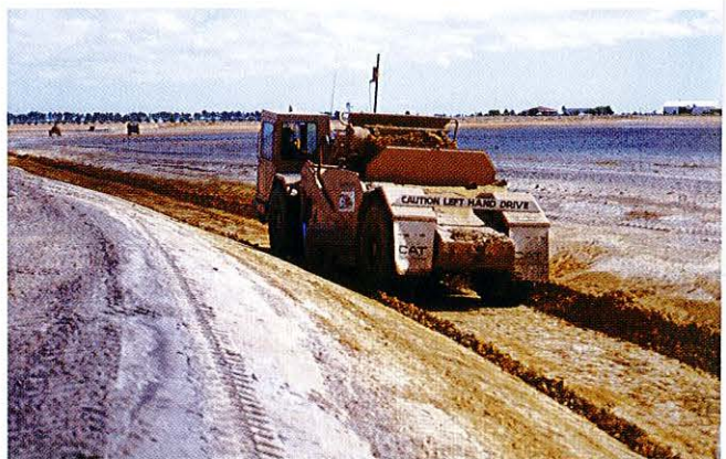
Photo 7.4 Excavation of a surface drain.
