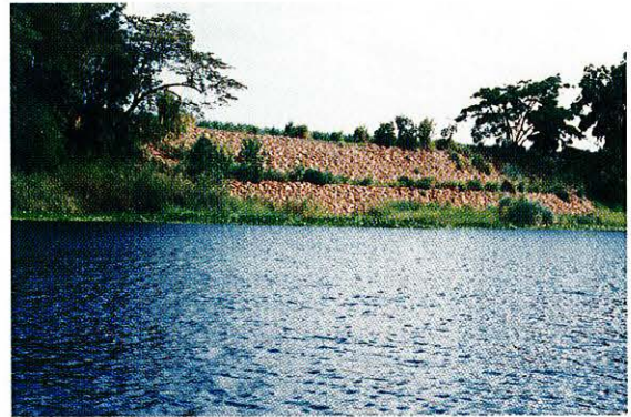
Rock revetment on the Herbert River: note gap in riparian vegetation
