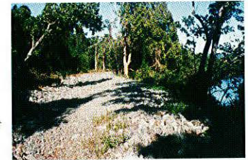
Rock spillway on Herbert River near Ingham
