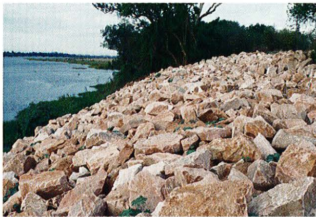
Plate 1.8 Traditional hard engineering in streams: Rock revetment on the Burdekin River
