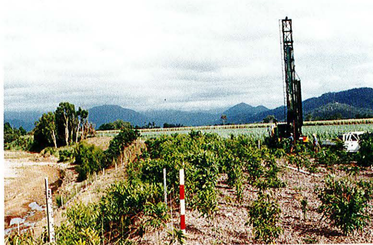
Plate 3 Trial stabilisation works; Treatment 1 in the foreground
