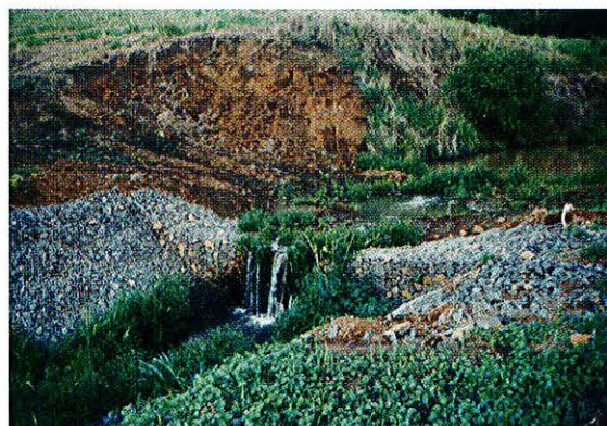
Rock gabion drop structure on Rankin Creek (Atherton Tableland)
