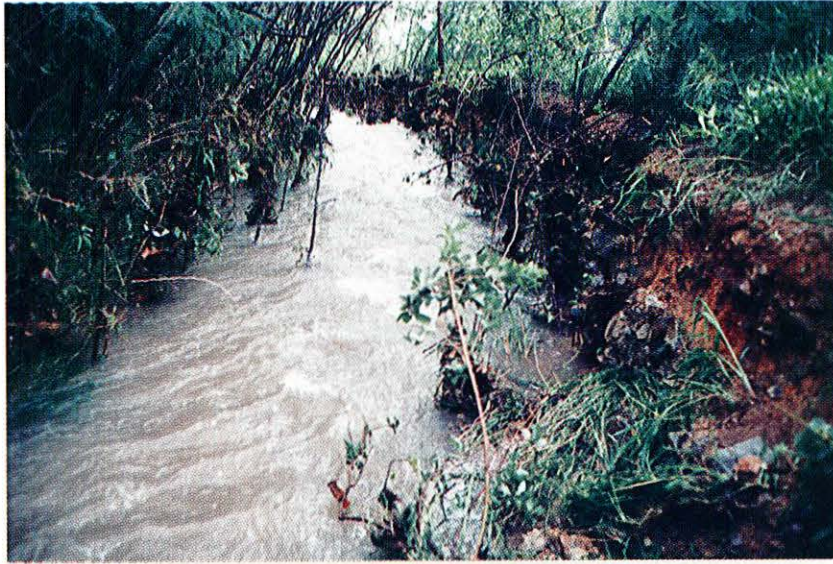
Plate 2.7 Fluvial bank erosion
