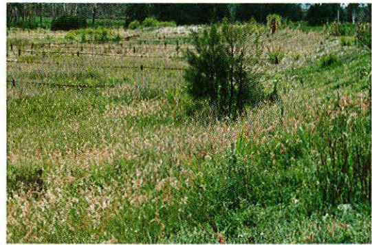
Steel pile and wire mesh embayments on Cattle Creek near Mackay
