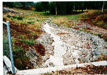
Grouted rock chute on urban stream in Townsville
