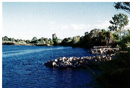
Rock Groynes on the Houghton River near Giru
