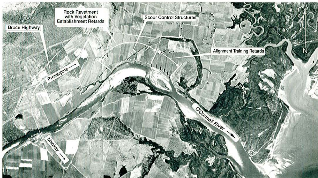
Plate 1 O'Connell River Study Site Locality Plan Source: Sunmap aerial photo, Calen 1989, Run 2, Nos. 61 and 63
