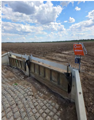
Figure 6: ABOVE: Automated winch driven controller. RIGHT: Direct drive removable controller.
