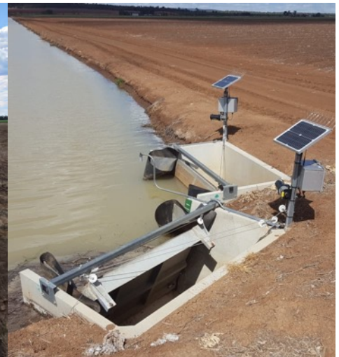
Figure 6: ABOVE: Automated winch driven controller. RIGHT: Direct drive removable controller.
