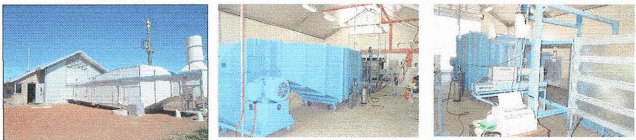
Figure 2. Pesticide Wind Tunnel Research Facility.
