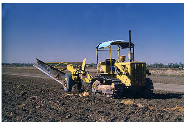
Channels may be regularly re-shaped and de-silted with excavators, graders, and delvers, effectively controlling weeds.
