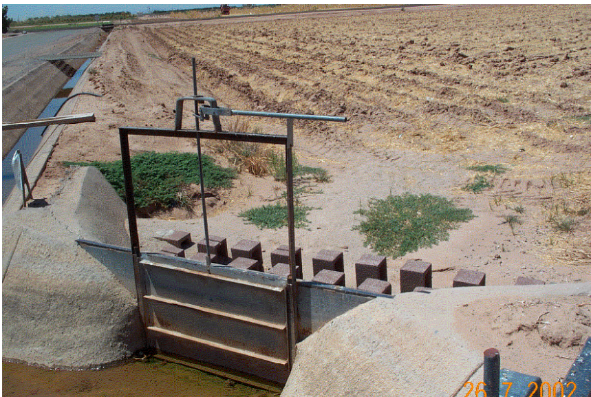
Plate 3: Modifications to allow rapid application of irrigation water to field and minimise soil movement. Note channels are concrete.
