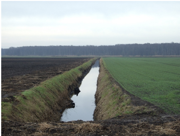
Figure 10 A typical landscape in “The Fens”. In summer, these drains are blocked and used to sub-irrigate the neighbouring fields.
