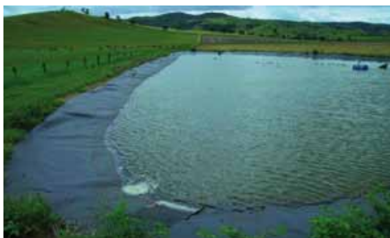
Seepage and evaporation mitigation measures in place on a farm dam
