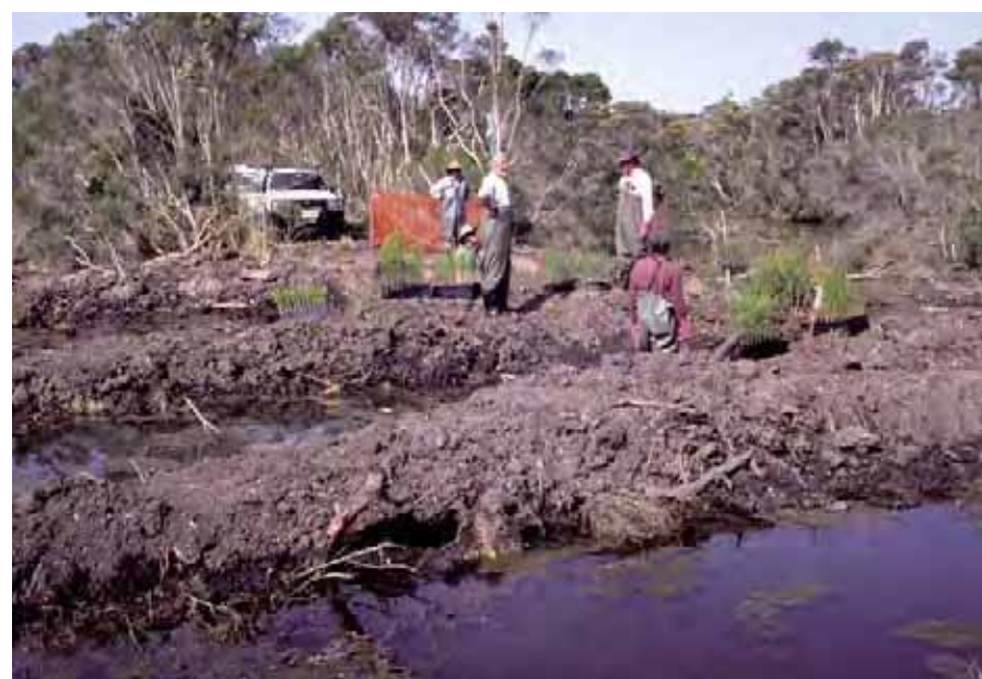
Figure 12.4: Artificial earthen hummocks used for the fourth revegetation trial. Twelve rows of hummocks were created, each ~ 15 m long x 1 m wide x 0.5 m high.
