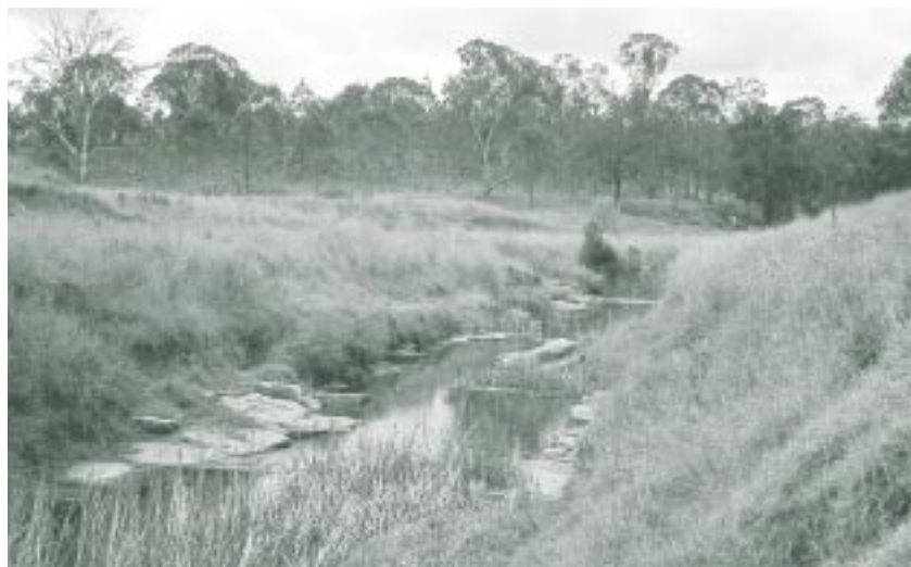
Emu Creek. Excessive clearing and heavy livestock traffic has severely degraded the streambanks and riverbed.
