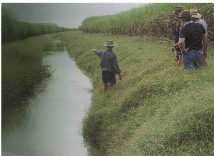
Figure 8.23 Thick growth of Pangola grass planted on the right bank by the property owner, acts as a filter strip for runoff from the field and protects the drain bank, while the unprotected left bank erodes.
