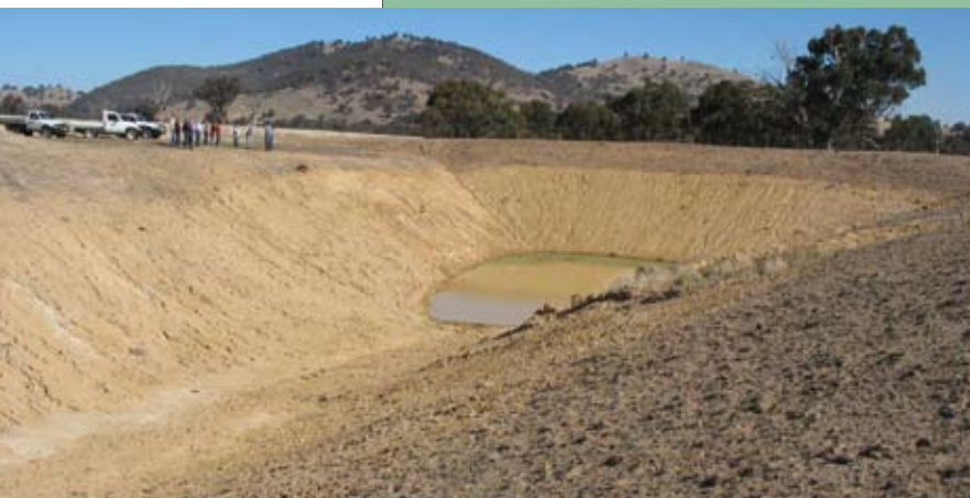
A dam built at the head of a gully as part of treatments being tested on the site.
